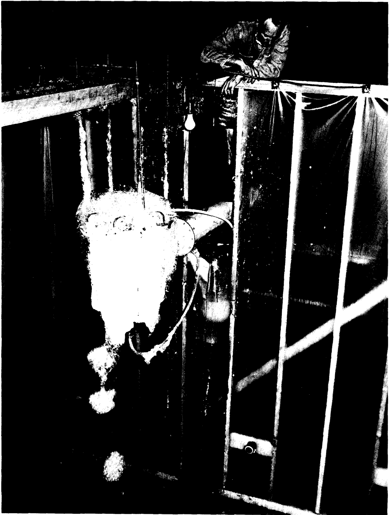
Figure 19. Generator installed at the 30 foot level; the generator plate housing was cut away to allow free foam flow.
