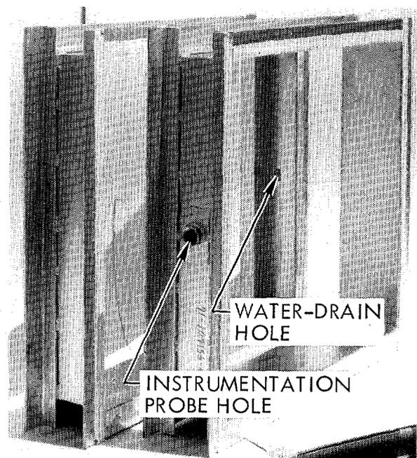
Fig. 10. Six-in. duct sections.
