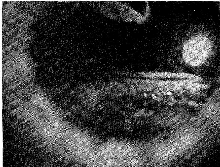
Figure 5. High-expansion foam was carried down the exhaust duct through the washer and half filled the filter housing.
