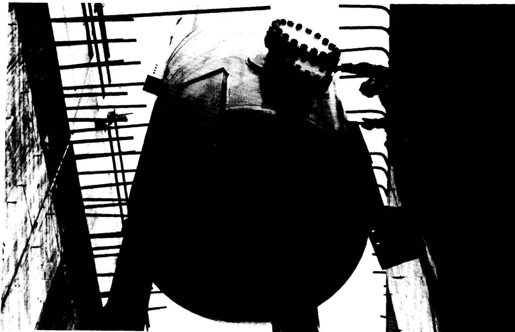
FIGURE 3 VERMONT YANKEE NUCLEAR POWER STATION VERMONT YANKEE ADVANCED OFF GAS SYSTEM Installation Of Absorber Tank TK 101-1G.
