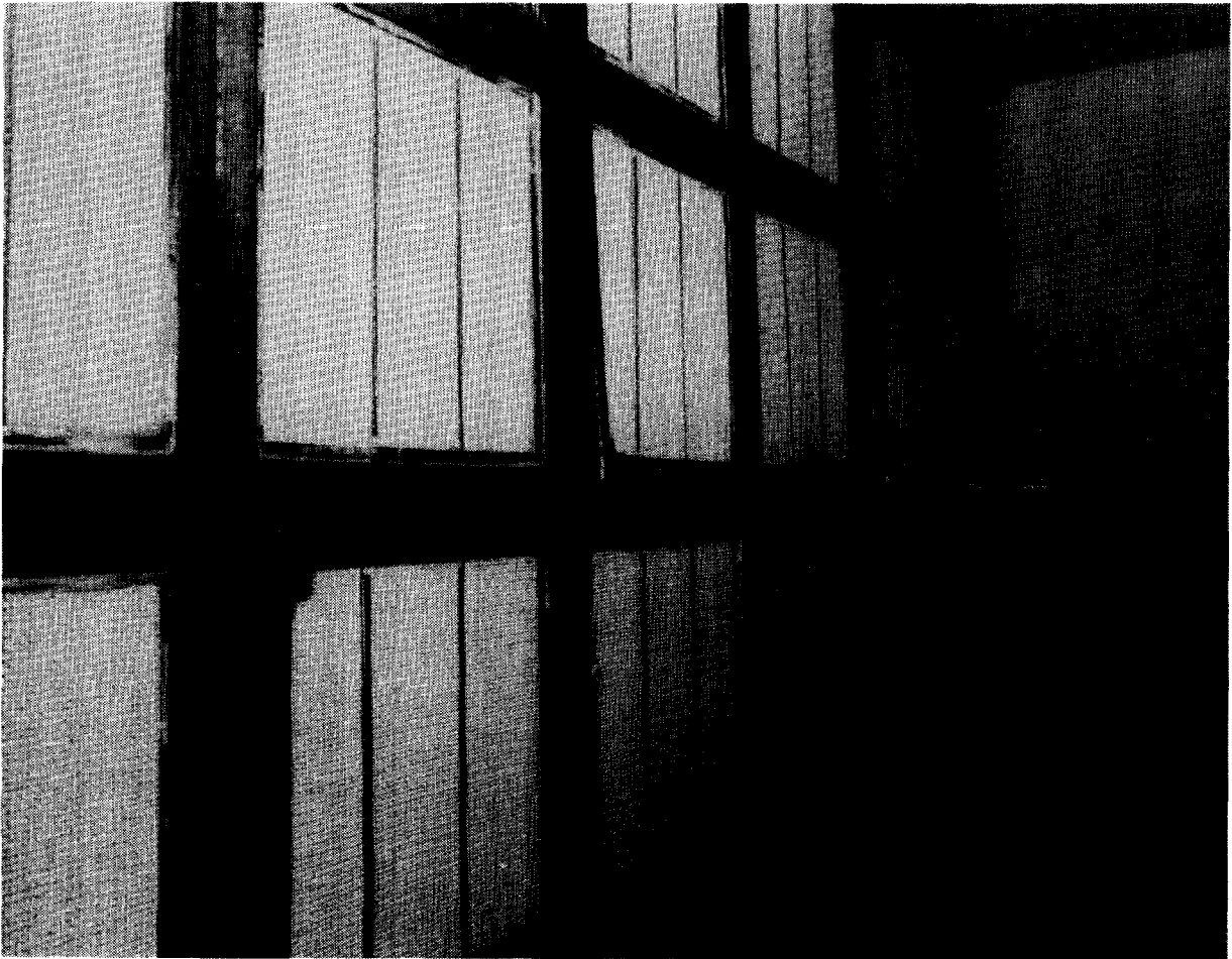
HEPA FILTER SYSTEM AFTER CONVERSION TO FLUID SEAL WITH DOP DISTRIBUTION SYSTEM INSTALLED
