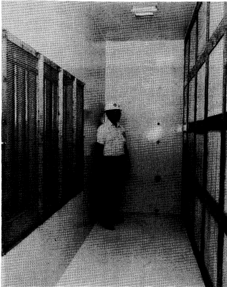
Exhaust Grill And Downstream Side Of 2nd HEPA Filter Bank
