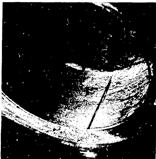
FIG. 2 CORROSION CAUSED BY IODINE AT A UNHEATED PIPE FLANGE OF THE PASSAT FACILITY
