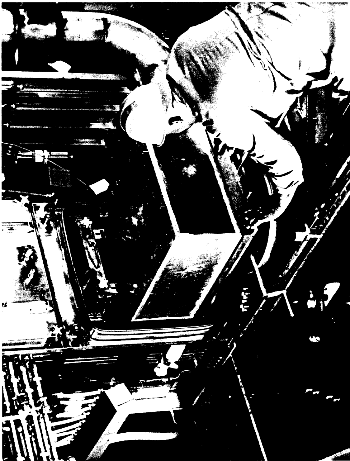
Figure 21 Cleanable steel filter being inserted into filter housing.
