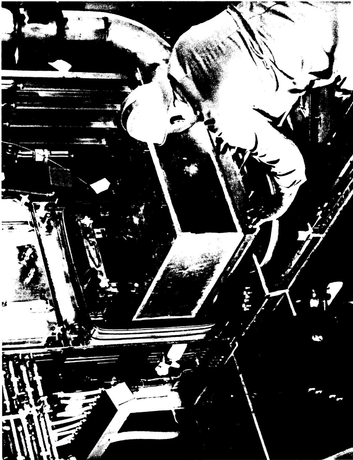
Figure 21 Cleanable steel filter being inserted into filter housing.
