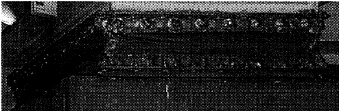
Figure 4 - Example of Potential Leak Point (flexible connection)
