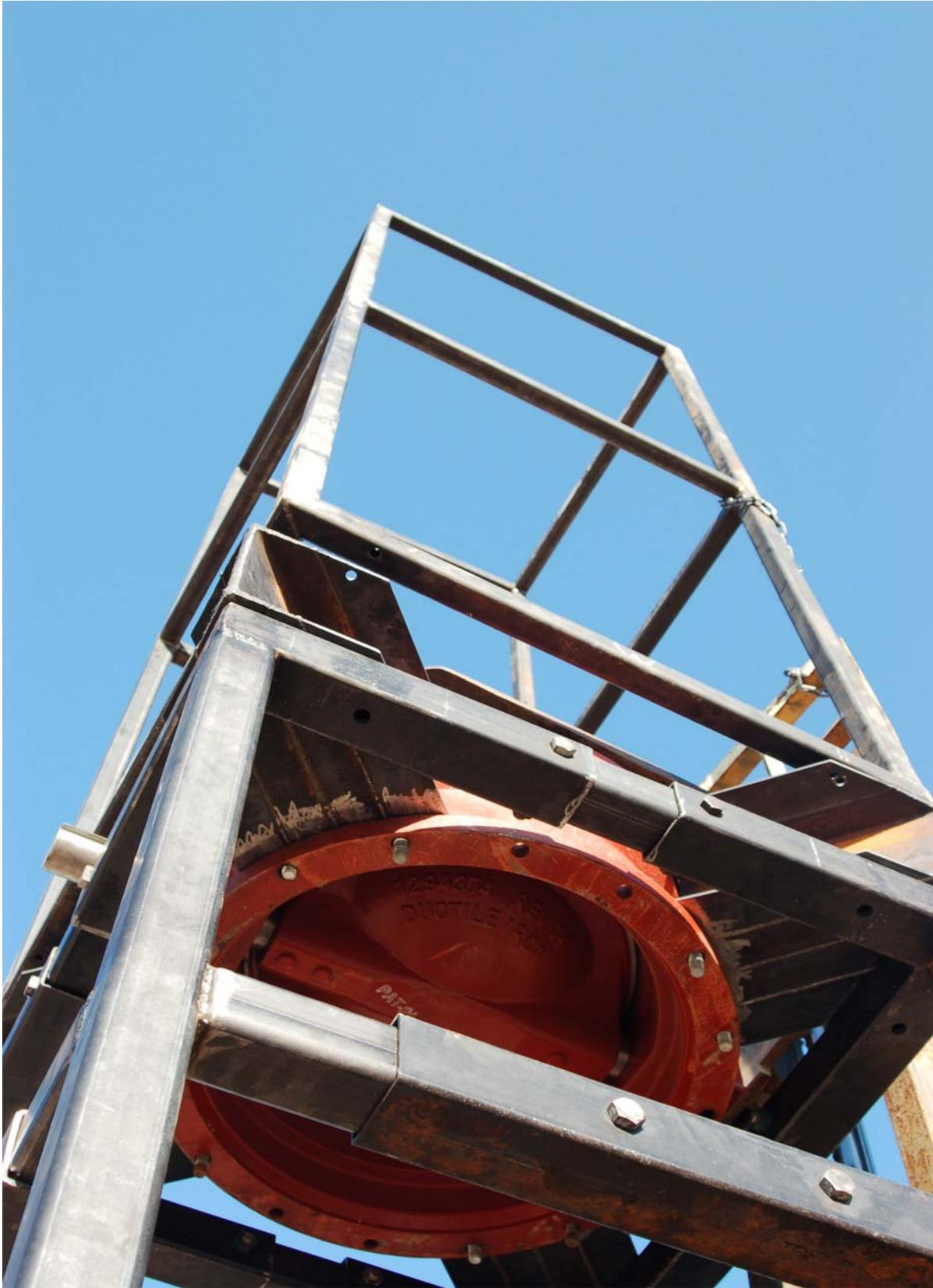
Figure A-4: Bottom view of preliminary assembly of valve support structure, valve, and upper pipe-enclosure cage.
