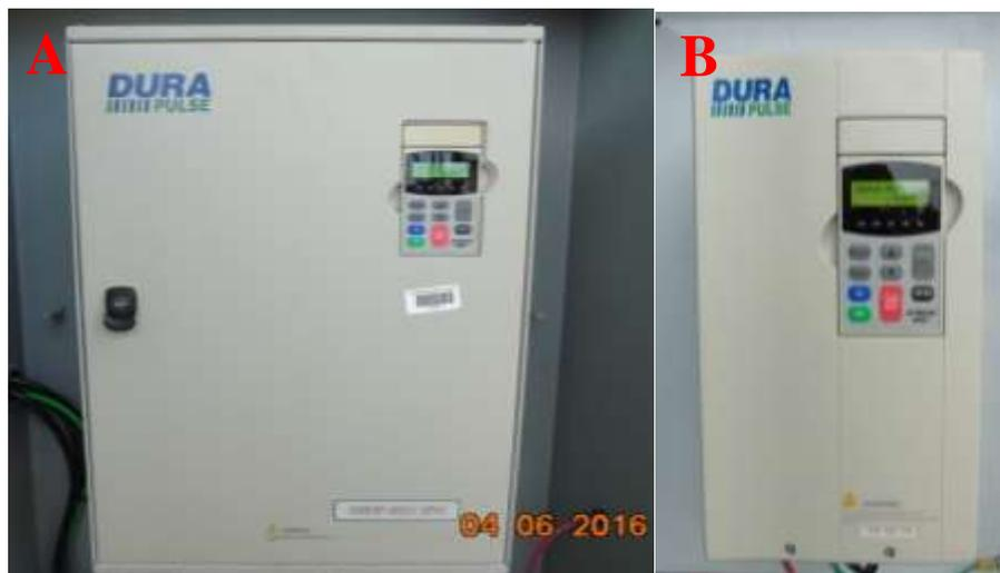
**Figure 5.** Photo of the variable speed drives for the fans on the RLSTS. A.) Large fan. B.) Small fan.
