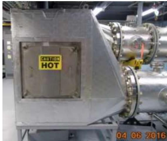
**Figure 4.** Photo of the safe change filter housing on the RLSTS.
