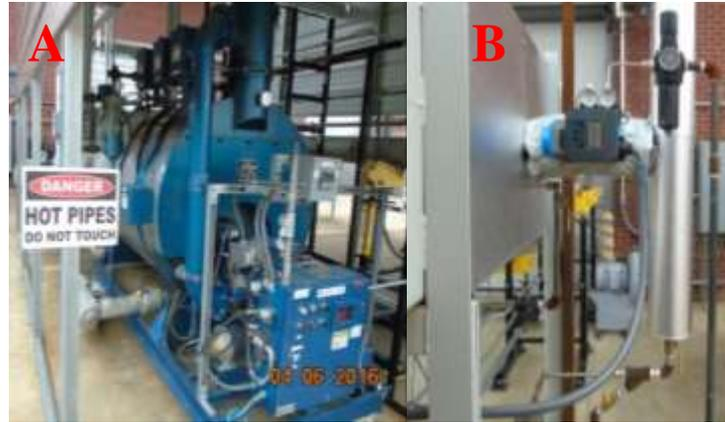
**Figure 10.** A.) Boiler. B.) Steam injection valve on the RLSTS.
