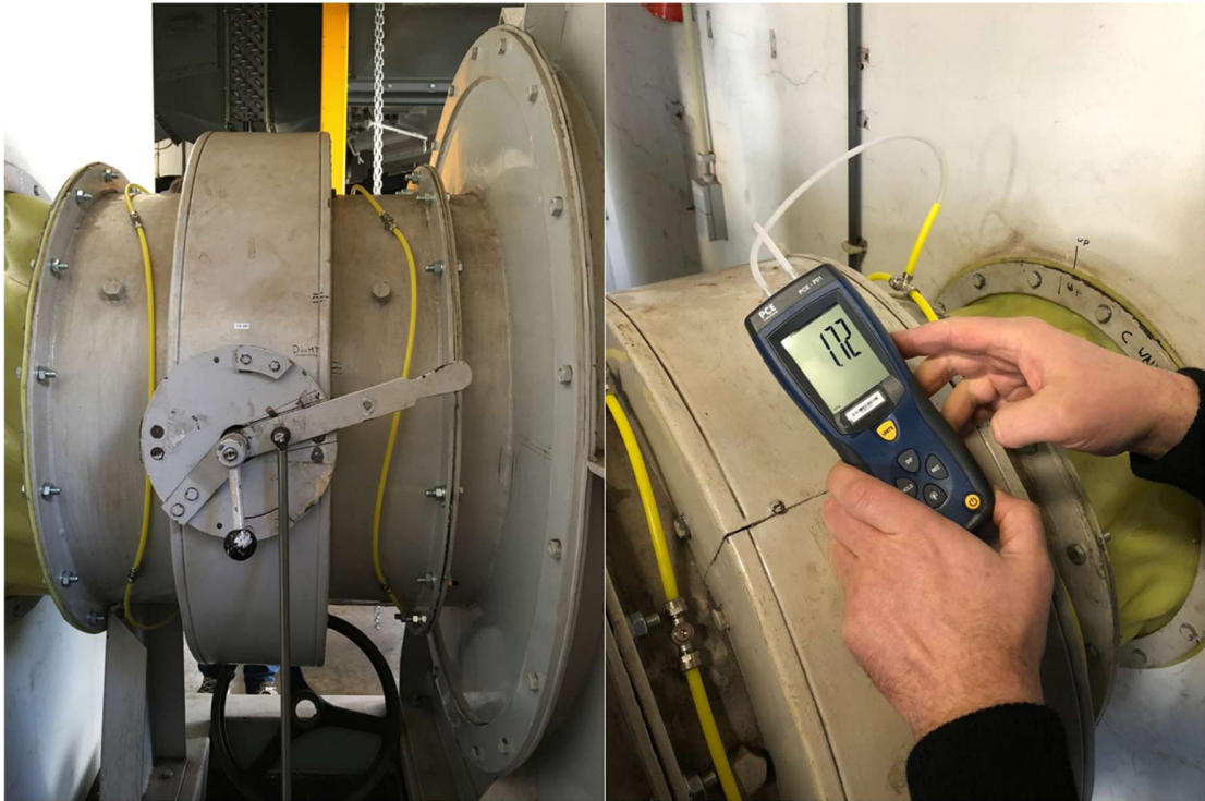
Figure 4 dp measurement taps installed and dp measurement being performed
